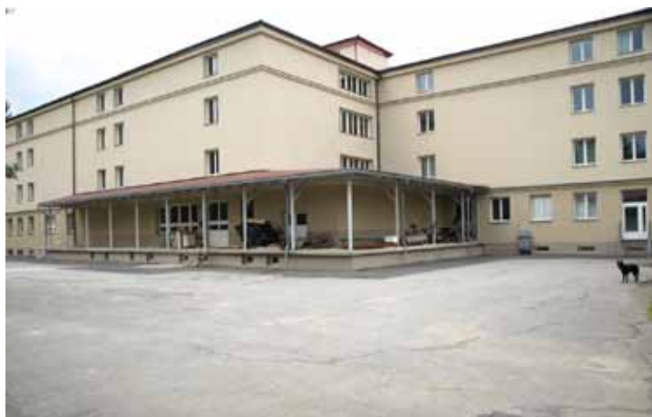
Ryc. 1. External view of the workshop building from with leading ramp
